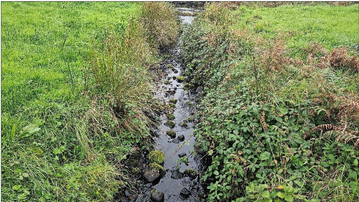
Plate 3.46 Representative image of site D29, September 2023
