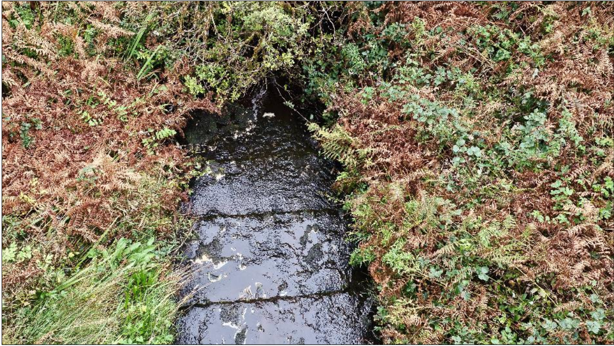
Plate 3.41 Representative image of site D24, September 2023
