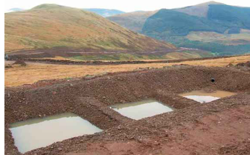
Example of constructed in-line silt traps
