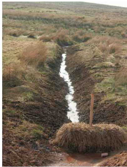
Straw bale temporary silt trap
