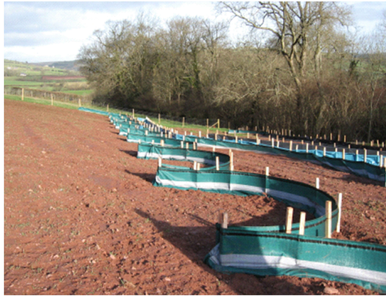
Example of installed silt fencing
